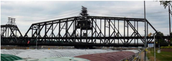
The Rock Island Arsenal Government Bridge, built over the Mississippi River in 1896 between Rock Island, IL and Davenport, IA, is just one of over two hundred bridges owned by the United States Army. Dr. Giles placed dozens of sensors on this bridge and used the sensors to objectively monitor the bridge's stability.
